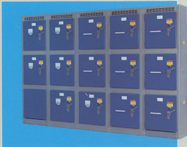
Multi-zone SCR power center for lehr heating element control.
